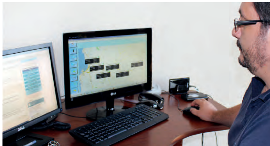
An operator at JVRE's headquarters using SCADAConnect to monitor flows
