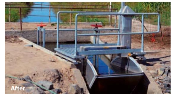
Operational spills are eliminated and upstream pool level is maintained
